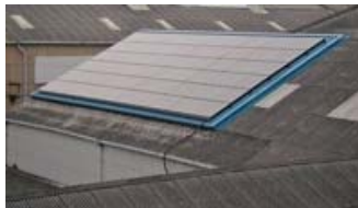
[太陽光発電10KWを設置]
