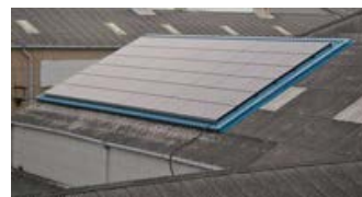
[太陽光発電10KWを設置]
