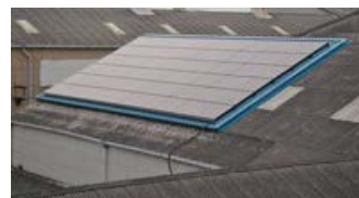
[太陽光発電10KWを設置]
